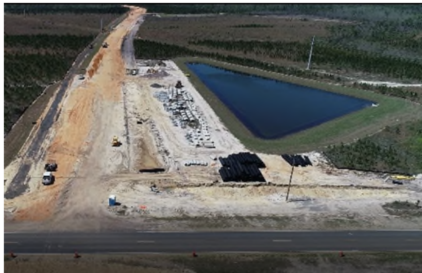
S.R. 370 (Gulf Coast Parkway) New Road Construction (District 3)
