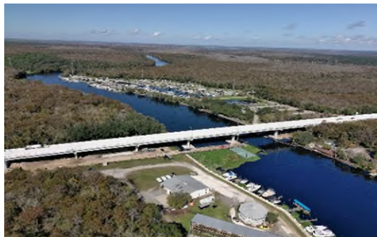
S.R. 44 Bridge (District 5)
