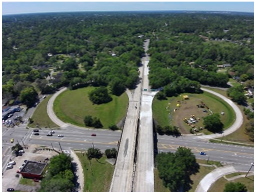
Emerson Expressway Resurfacing and Rehabilitation (District 2)
