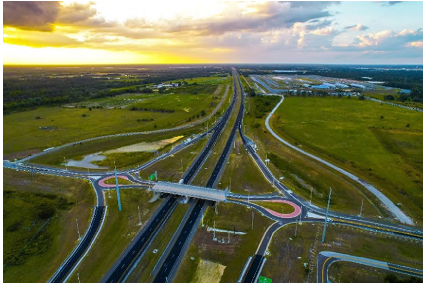
Polk Parkway Widening from Old Dixie Highway to Pace Road (Florida's Turnpike Enterprise)
