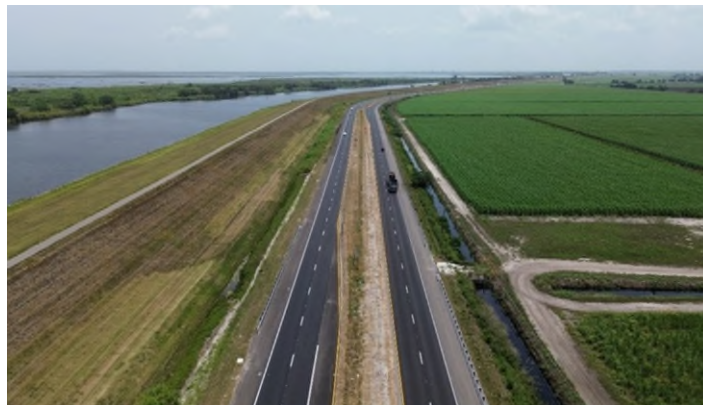
S.R. 25 / U.S. 27 Resurfacing and Restoration (District 4)
