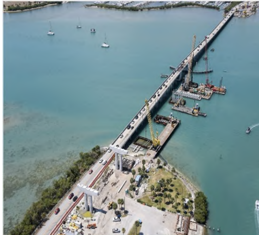
S.R. AIA North Causeway over the Intracoastal Waterway (ICWW) (District 4)
