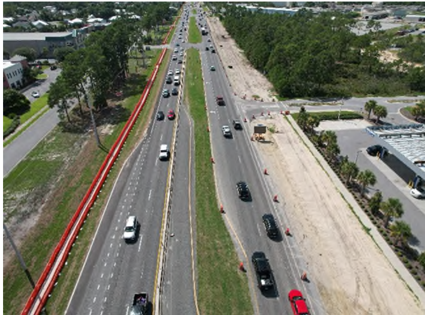
U.S. 98 (Panama City Beach Parkway) Widening (District 3)
