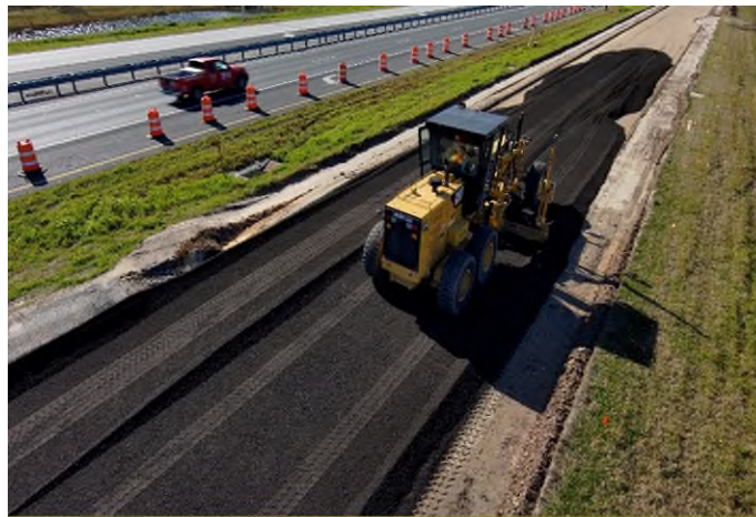
U.S. 301 Concrete and Asphalt Test Roads (District 2)
